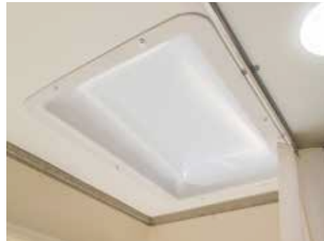
Skylight over Tub
