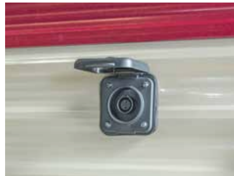
Solar Prep and Wiring
